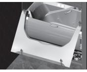
Remove the outer wall of the bathtub by pulling the bottom of the apron panel outward.
