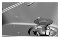
• Put the drain upside-down on a towel in the bathtub and make sure not to break the drain supply lines.
